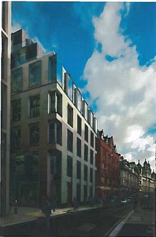
Endurance Land is working with Scottish Widows to refurbish 35 Chancery Lane
